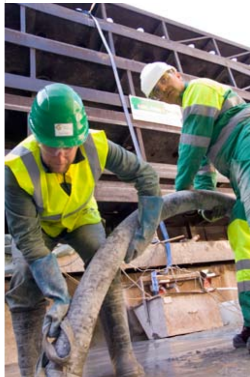
Coulage de Ductal®, béton ultra haute performance Lafarge.
